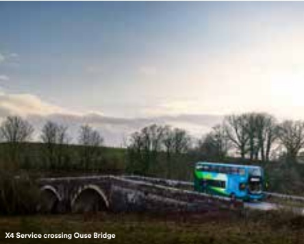
X4 Service crossing Ouse Bridge
